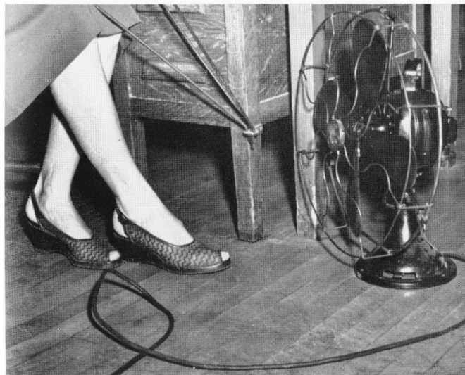
Here's a wall-type fan set on the floor where it was never meant to be used. Fans like this should not be on floors or under desks (yes, some people even put them there) unless they are in mesh boxes. It is a hazard to feet, fingers and clothing — and a tripping hazard.
